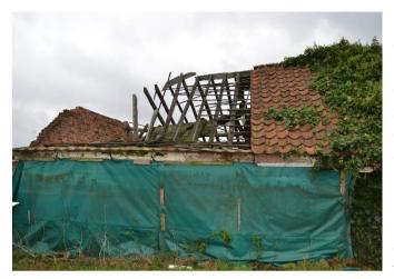
Repair to the northern wall will gable required where this was damaged when the cart shed roof collapsed. It is observed that the collapse was due to the poor condition of the roof as a result of rot and infestation of the timbers and through no failure of the walls or foundations
