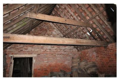
with collars providing lateral support to the wall plates and preventing roof spread. As with all timber roof structures on traditional barn buildings, it will be necessary to undertake repairs the to roof
