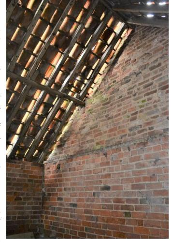
support allowances for snow loading and dead loads including existing pantiles and to support new loading required for the conversion. This includes new dead loads including standard services, insulation, and new internal finishes. It is
