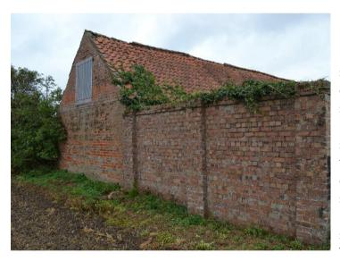
ln general, the brickwork appears to be in good condition, showing no obvious evidence of any significant structural movement, although minor some has fracturing occurred and there is some relatively minor misalignment of the southern gable wall. These minor fractures
